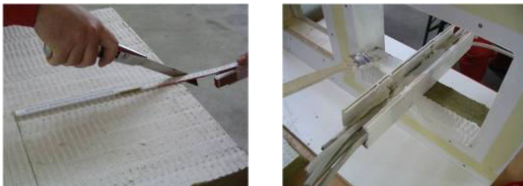
Figure 85: Cut to size of mineral fiberboard and coating of boards and reveal, source: Würth company
