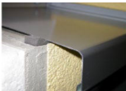
Figure 53 Horizontal joint under window sill towards facade surface with permeable sealing tape. Can also be executed in open form Source: [Österreichische Arbeitsgemeinschaft Fensterbank]
