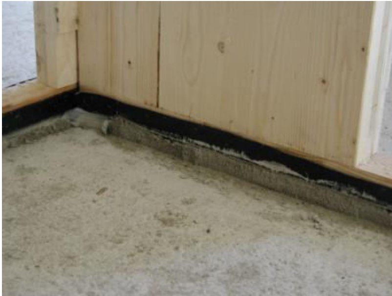
Figure 50: Support detail of an internal wall
