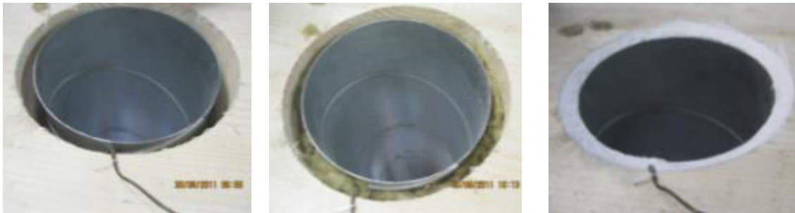
Figure 90: Insulation of the annular gap between ventilation pipe and wooden component with stone wool (center), application of an intumescent fire protection compound with a depth of about 15mm (right)
