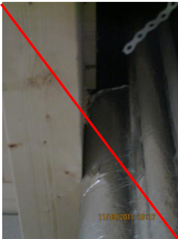
Figure 79: Incorrect execution: Due to a later extension of the shaft, non-combustible cladding of the wooden beam inside the shaft is not possible
