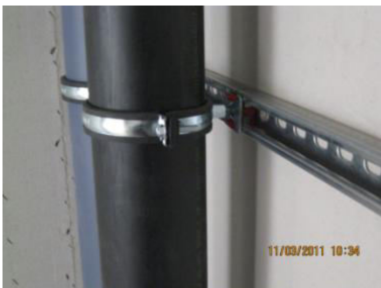
Figure 81: Sound protection decoupling of pipes
