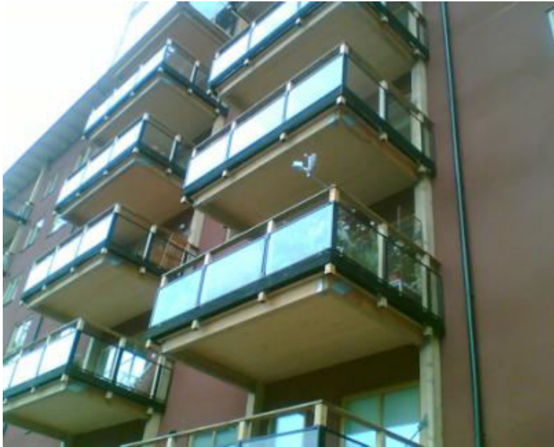
Figure 107: Prefixed balcony construction, source: Stora Enso company
