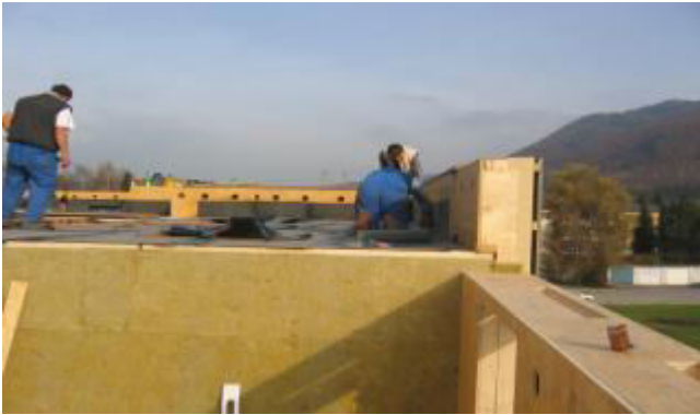
Figure 46: Vapor retarder (bituminous sealing) on a flat roof as a required weather protection
